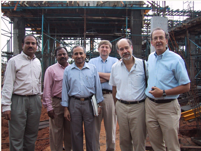
Building the vaccine facility at a nascent Bharat Biotech, in Hyderabad.
